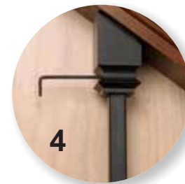
4 Snap shoe in place and tighten
